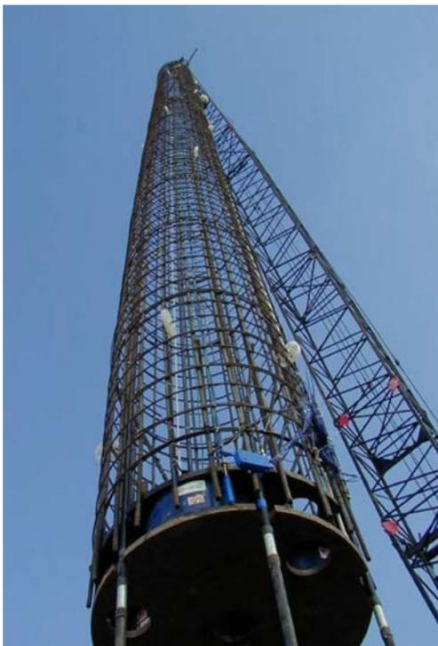
Figure 5.4 Load cell in reinforcement
